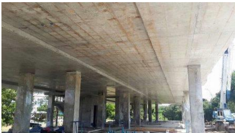
Fig. 1 Slab band system (Courtesy of Posteck Prestressing 2015)
